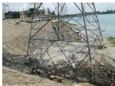
Placing tower on its foundation
