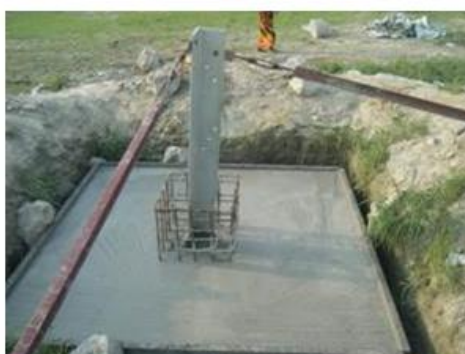
Casting CC into tower foundation
