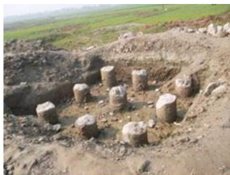
tower piling works
