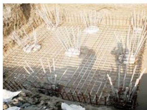
pile cap reinforcement
