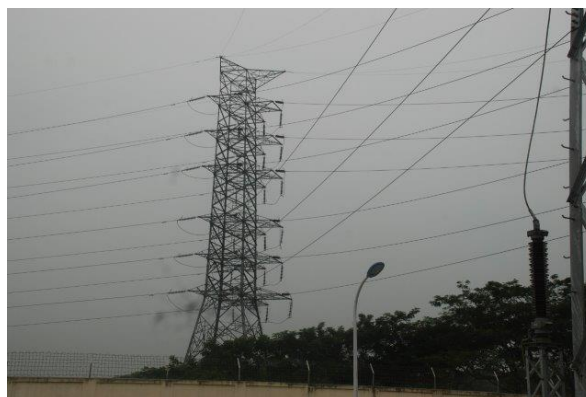
Picture 4. Double Circuit line-in line-out terminal tower
