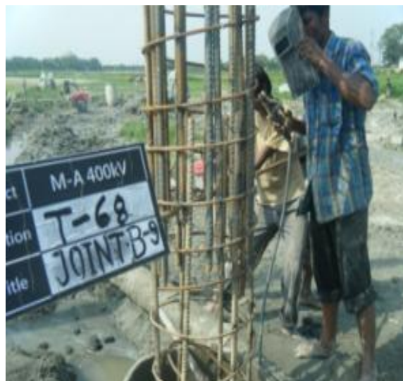
Figure 36: Welding of reinforcements
