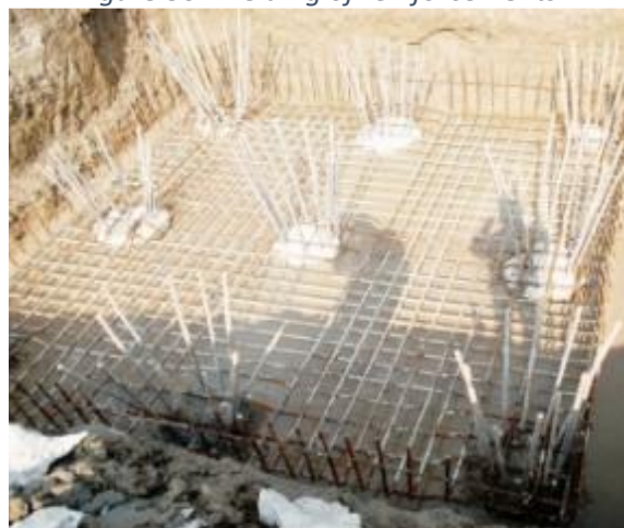
Figure 38: Pile Cap Reinforcement
