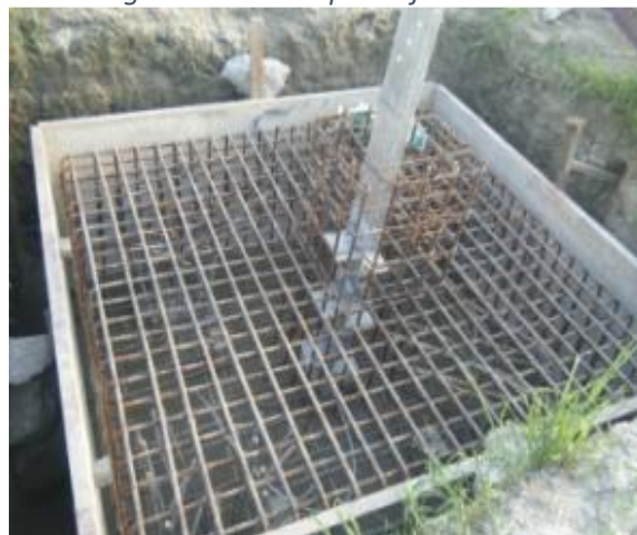
Figure 40: Providing detail reinforcements
