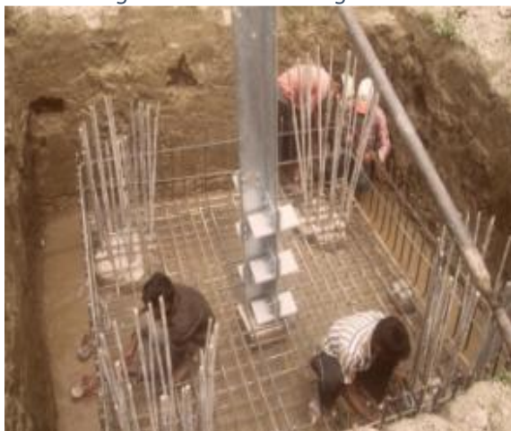
Figure 39: Striping the tower footing with steel
