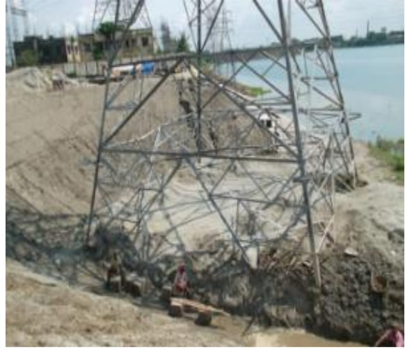
Figure 42: Placing Tower on its foundation
