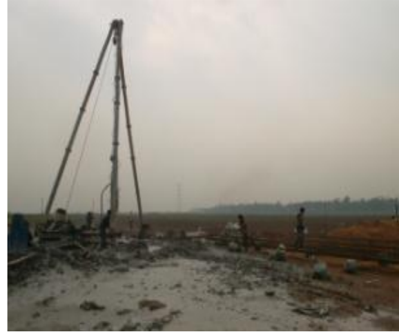
Figure 34: Piling Work
