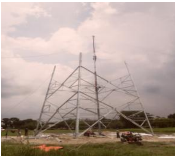
Figure 43: Tower Erection Work
