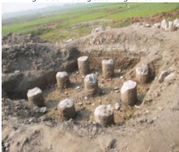
Figure 37: Tower Pilling Work
