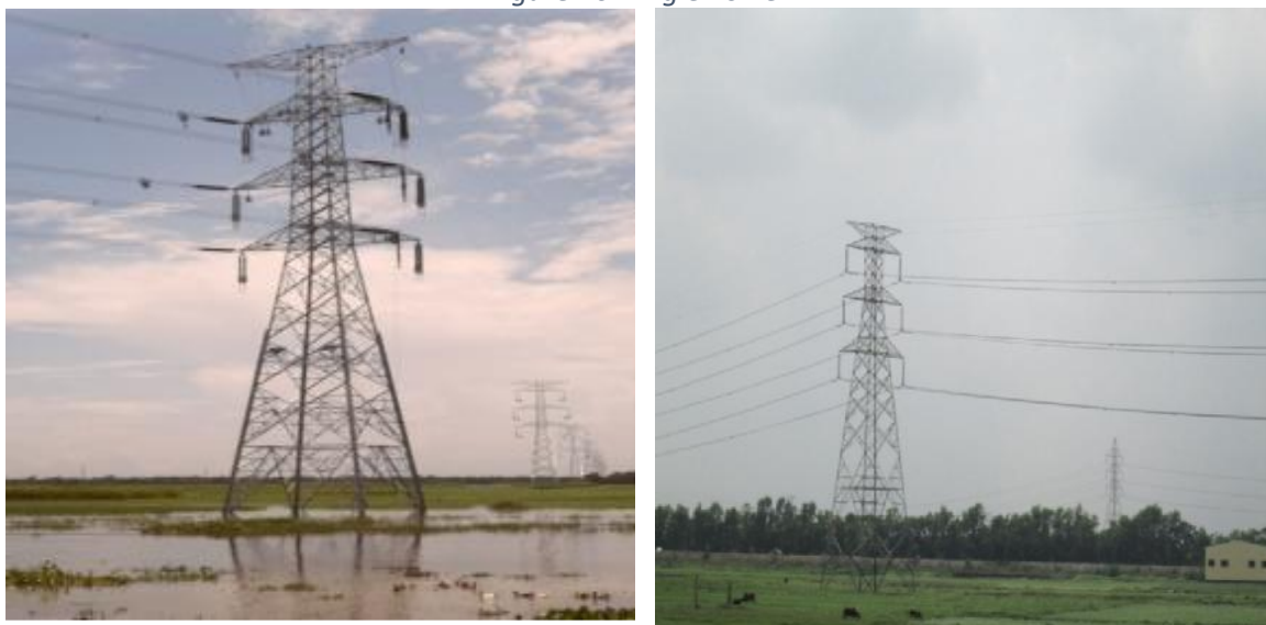
Figure 27: Suspension Tower
