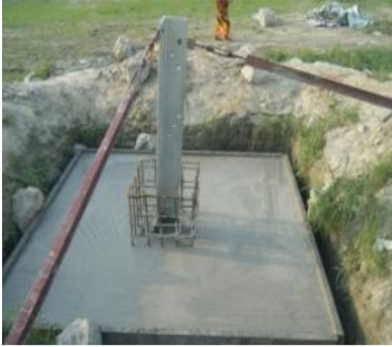
Figure 41: Casting CC into tower foundation
