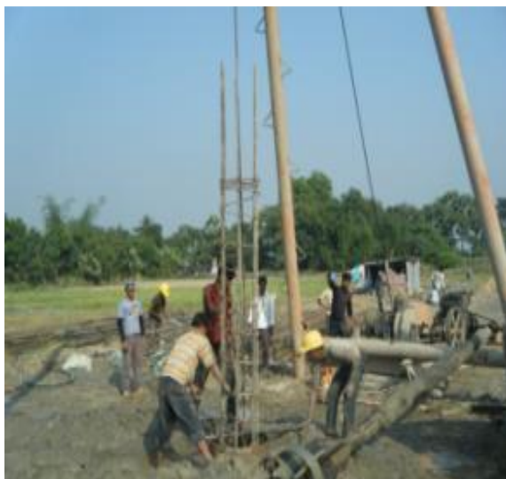
Figure 35: Placing steel ring bunds
