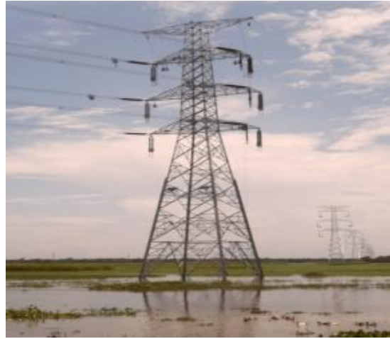
Figure 4.5: Suspension Tower
