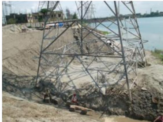
Figure 4.20: Placing tower on its foundation
