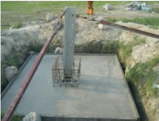
Figure 4.19: Casting concrete cement into tower foundation
