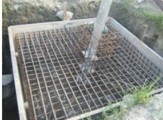
Figure 4.18: Providing detail reinforcements
