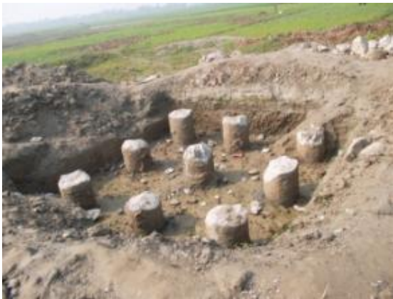
Figure 4.13: Placing steel ring bunds
