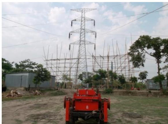
Figure 4.22: Conductor stringing
