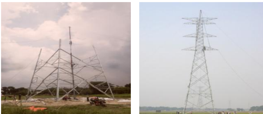
Figure4.21: Tower erection works
