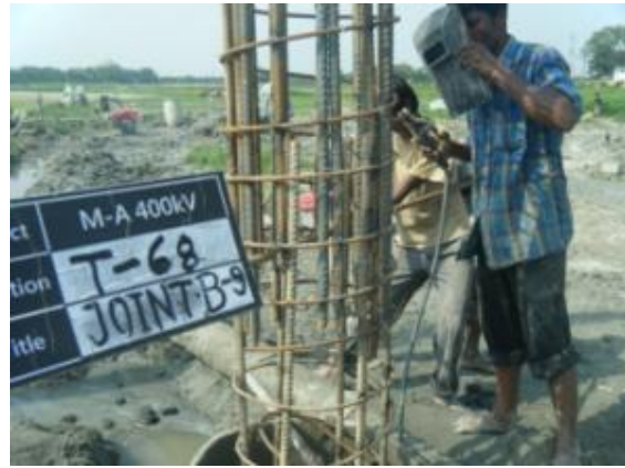
Figure 4.14: Welding of reinforcements
