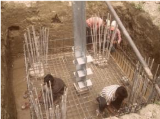
Figure 4.17: Striping the tower footing with steel
