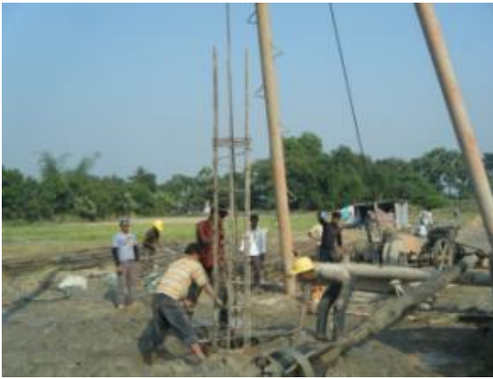
Figure 4.13: Placing steel ring bunds
