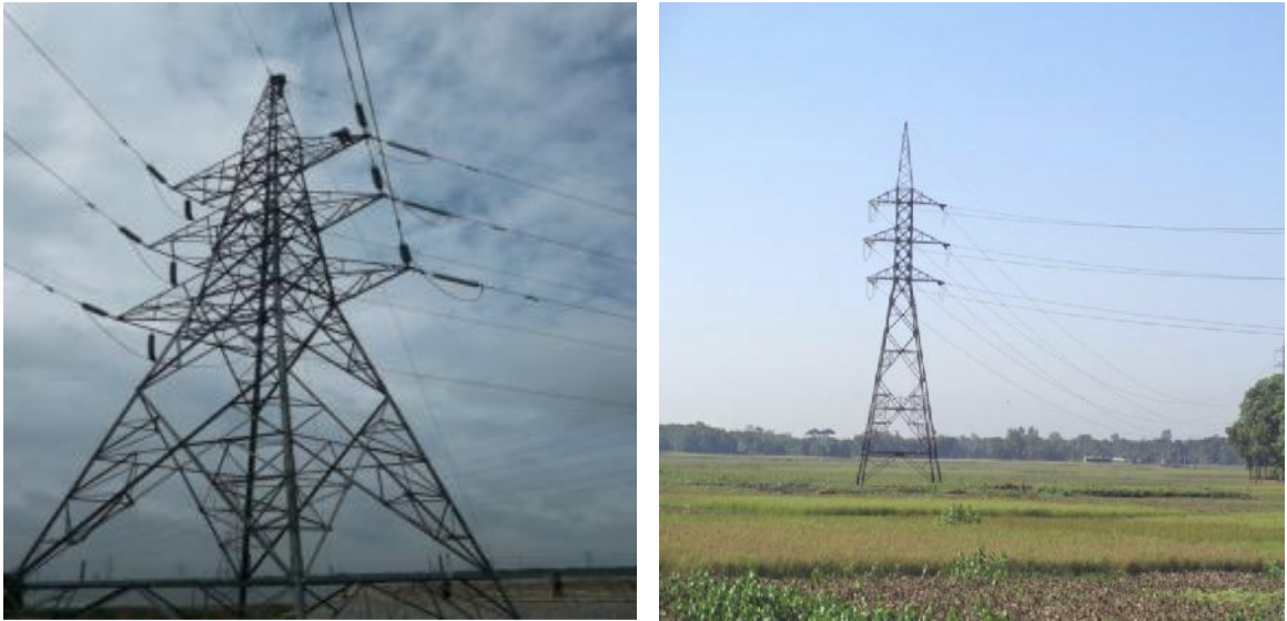
Figure 30: Angle Tower
