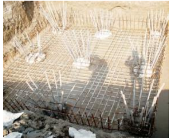
Figure 42: Pile Cap Reinforcement
