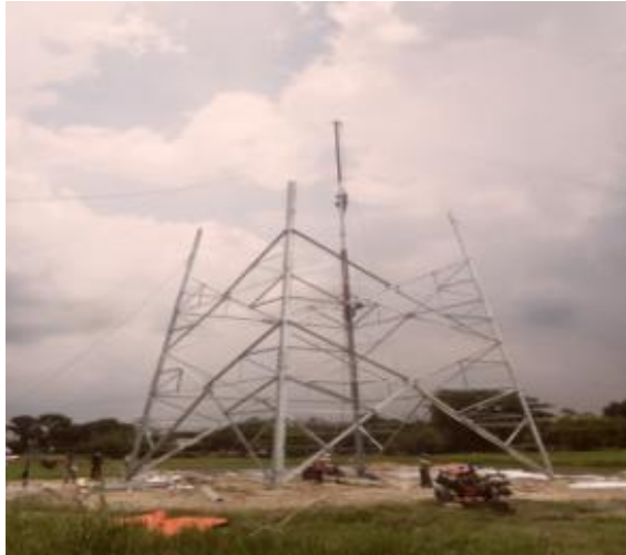
Figure 47: Tower Erection Work
