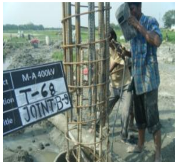
Figure 40: Welding of reinforcements
