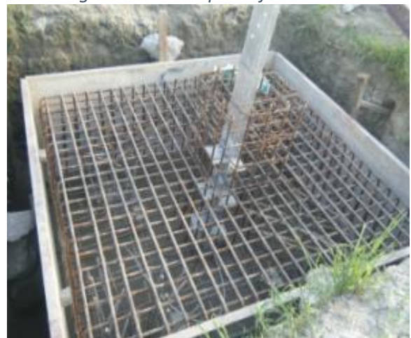
Figure 44: Providing detail reinforcements
