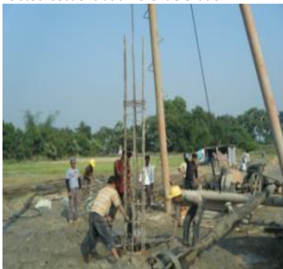
Figure 39: Placing steel ring bunds
