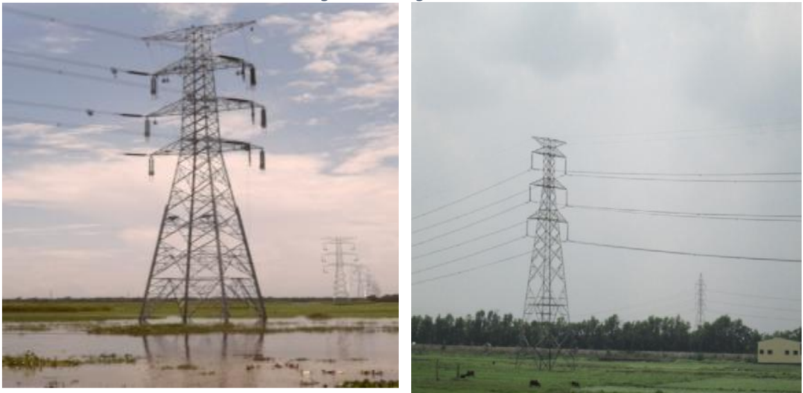
Figure 31: Suspension Tower
