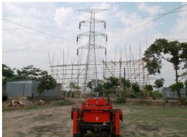
Figure 49: Conductor Stringing
