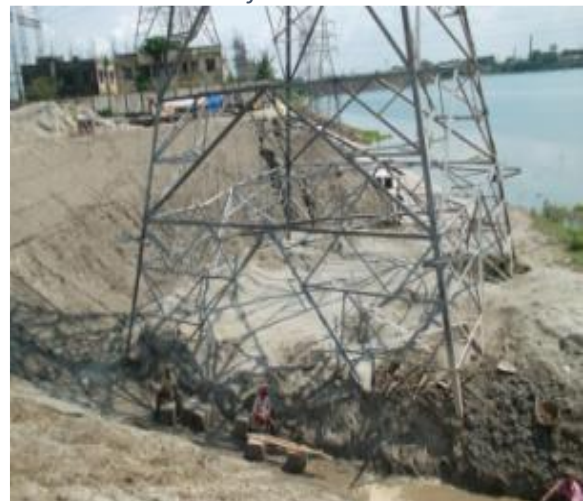
Figure 46: Placing Tower on its foundation
