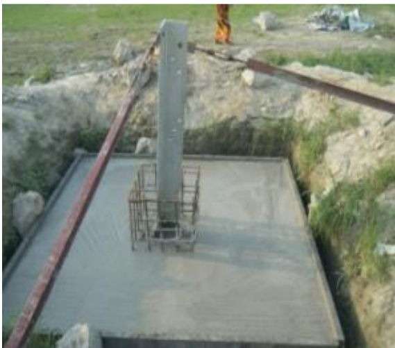
Figure 45: Casting CC into tower foundation
