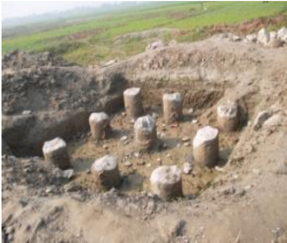
Figure 41: Tower Pilling Work
