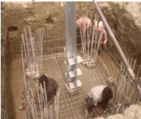
Figure 43: Striping the tower footing with steel
