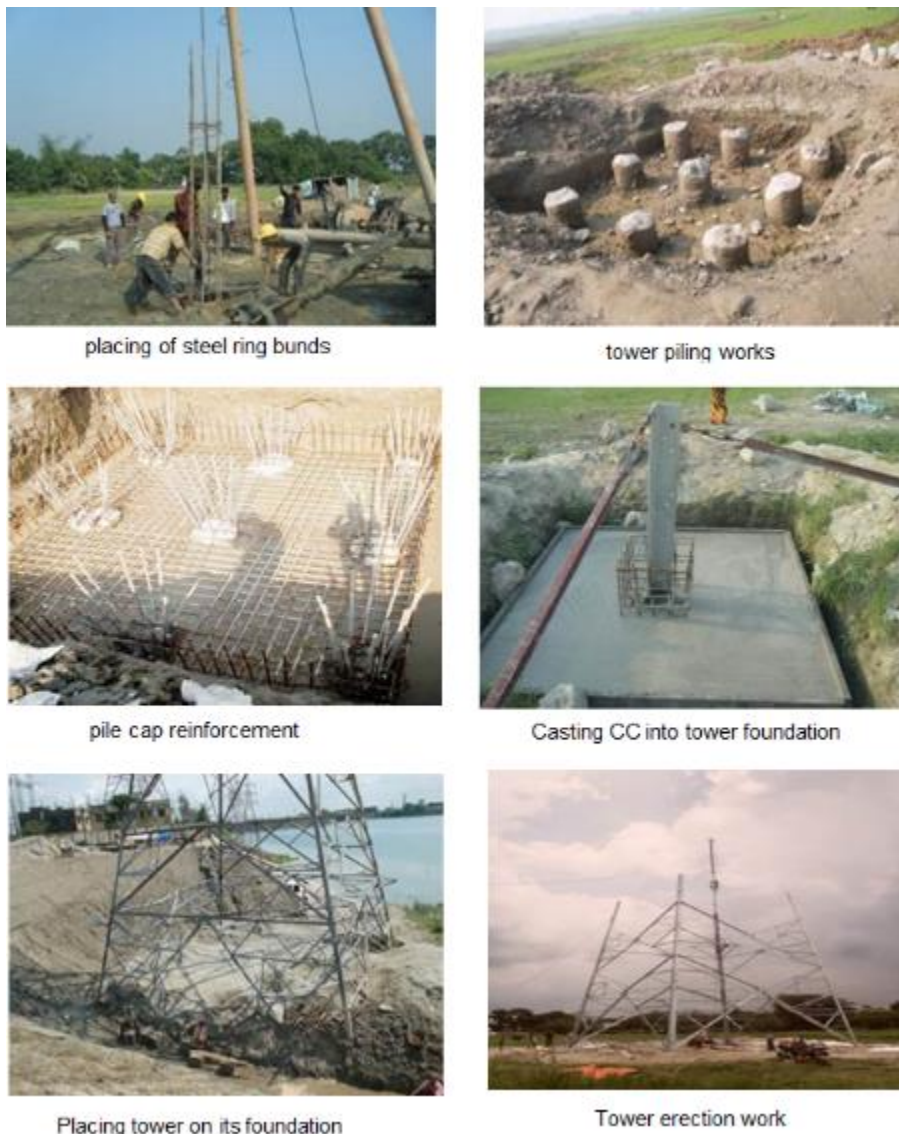
Figure 3-5: Associated Civil Works for Transmission Line Installation
