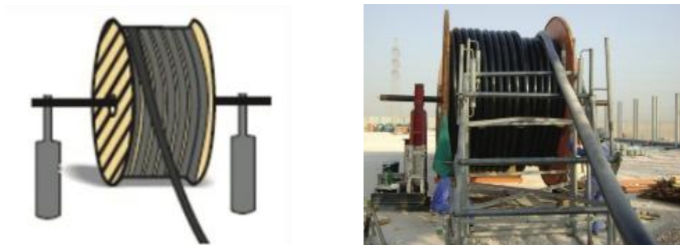
Figure 3-3: Placement of cable drum and correct method of pulling
