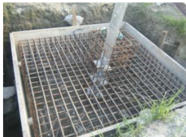
Figure 3.16: Providing detail reinforcements
