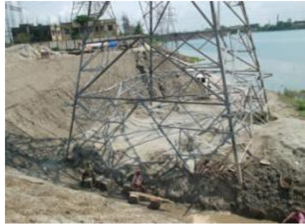
Figure 3.18: Placing tower on its foundation
