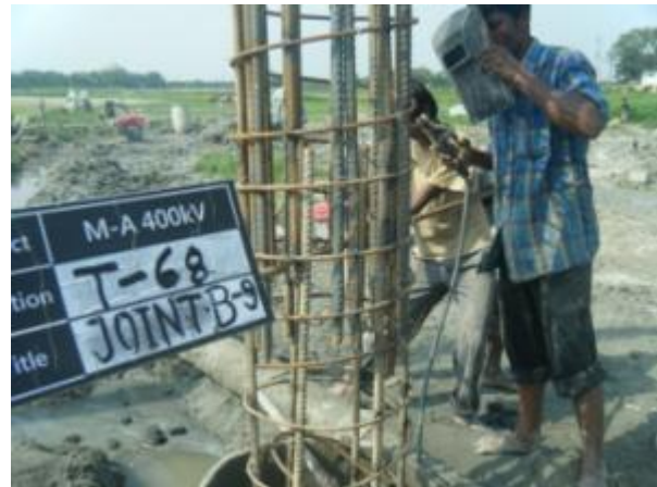
Figure 3.12: Welding of reinforcements
