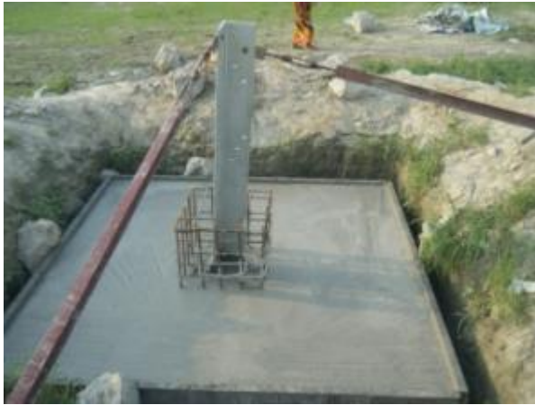
Figure 3.17: Casting concrete cement into tower foundation
