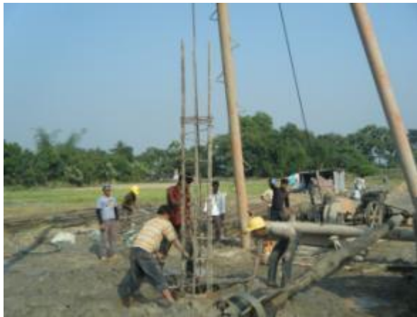
Figure 3.11: Placing steel ring bunds
