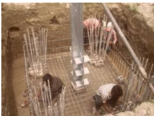
Figure 3.15: Striping the tower footing with steel
